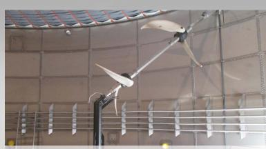
The double-propeller-agitator in the digester provides good mixing.
