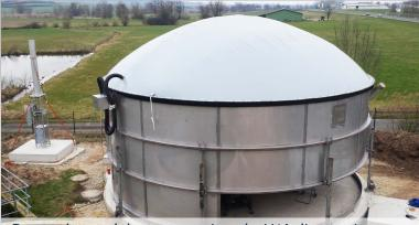
Due to the modular construction, the V4A digester is built within a very short time.
